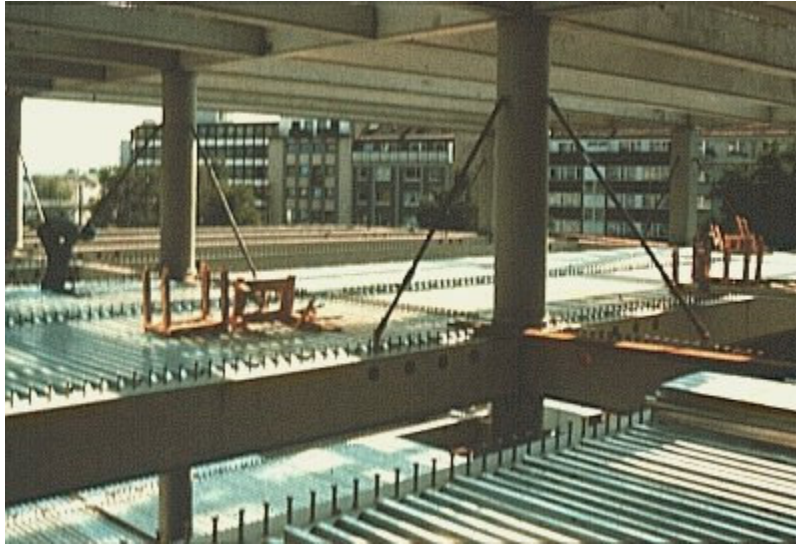
Picture 6 : The usual practice for commercial and industrial buildings is to construct the floors using metal decking which is embossed to provide composite action.
