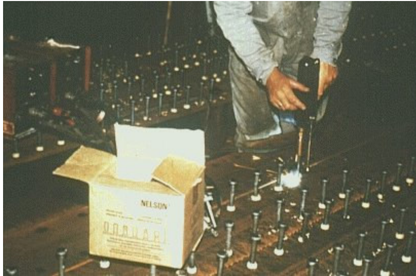
Picture 4 : Composite beams, subject mainly to bending, consist of a steel section acting compositely with one (or two) flanges of reinforced concrete.
