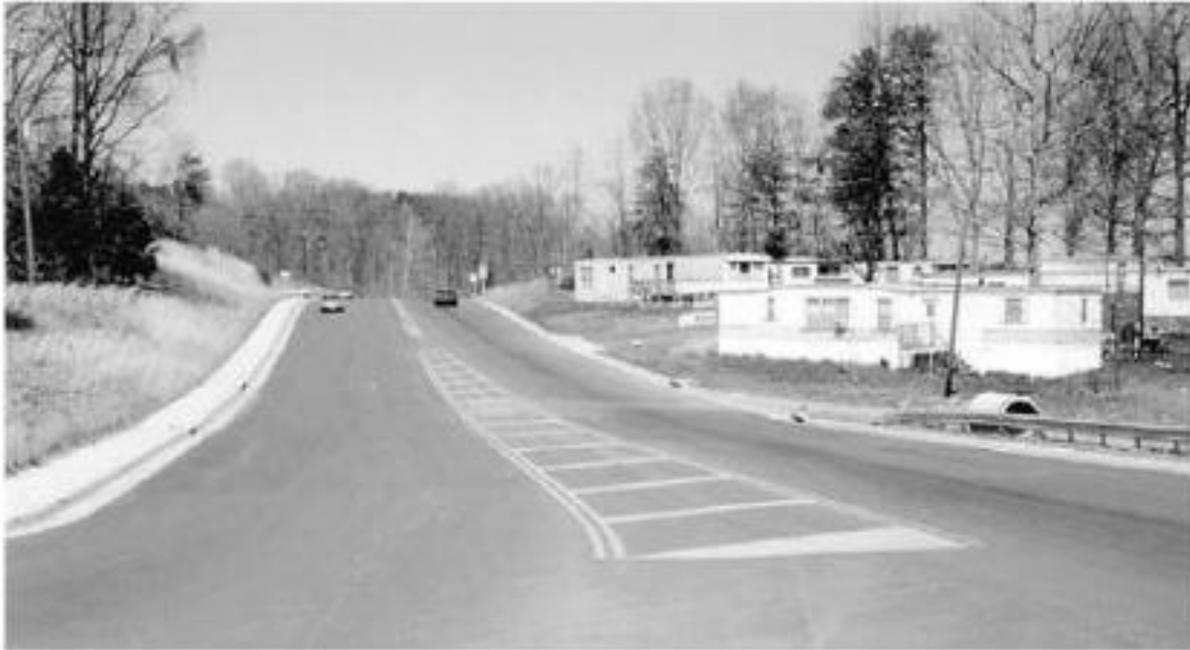
*Figure 43 Island Formed by Pavement Markings (Flushed Island)*
