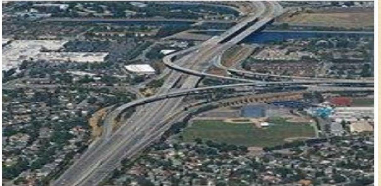
Figure 7 Three-Way Directional Interchange
