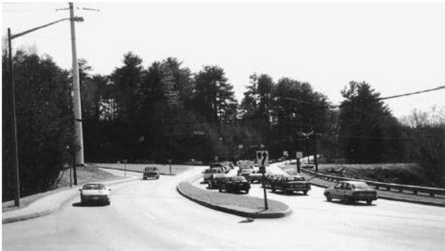
*Figure 42 Curbed Island at an Intersection*
