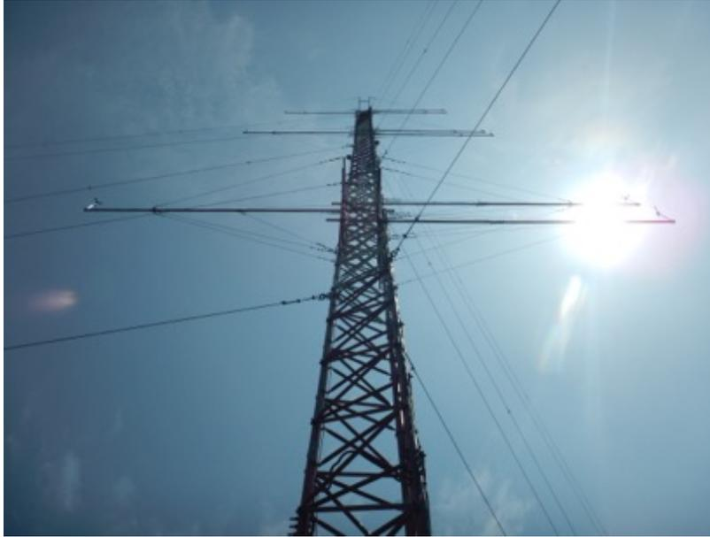
**Figure 12. Typical MET tower configuration with sensors attached to boom extensions.**
