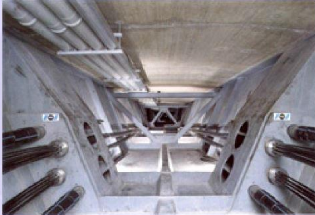
Figure 1-2.2 External prestressing of a box girder
