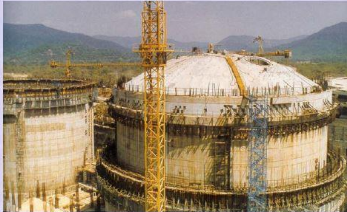
Figure 1-2.7 Circularly prestressed containment structure, Kaiga Atomic Power Station, Karnataka
