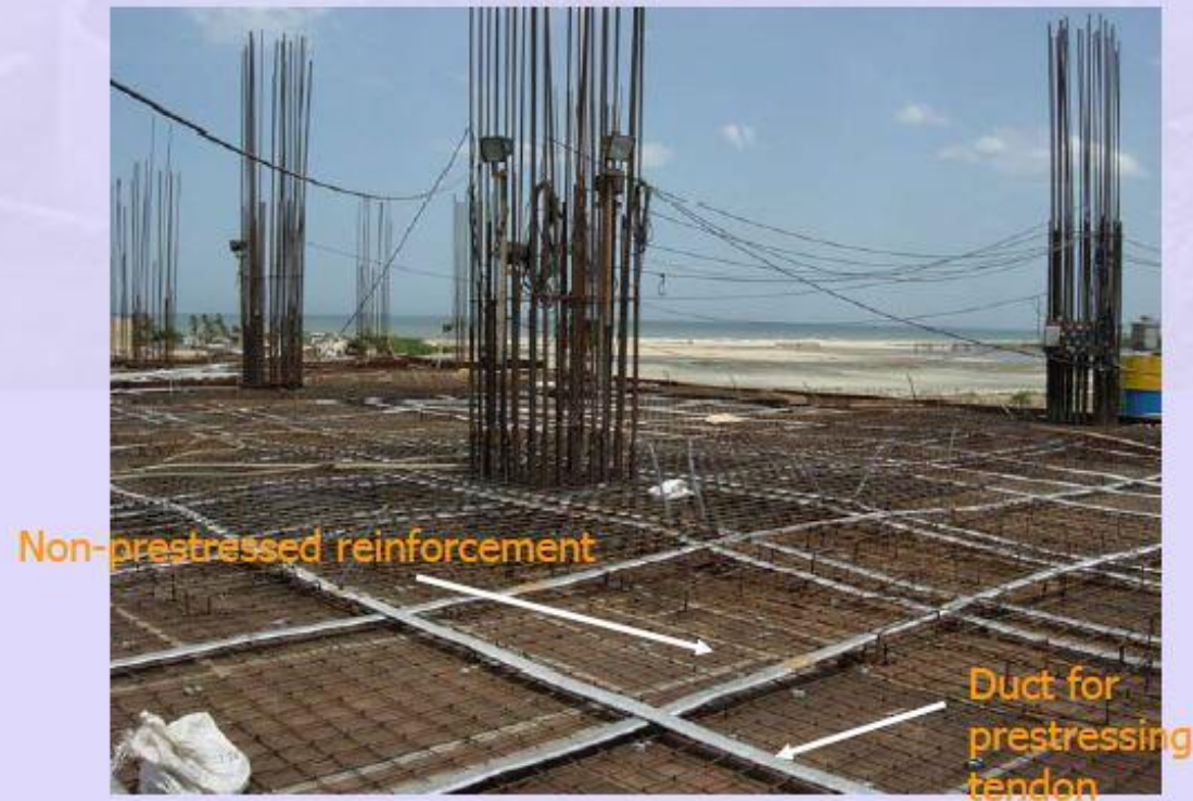
Figure 1-2.8 Biaxial prestressing of a slab
