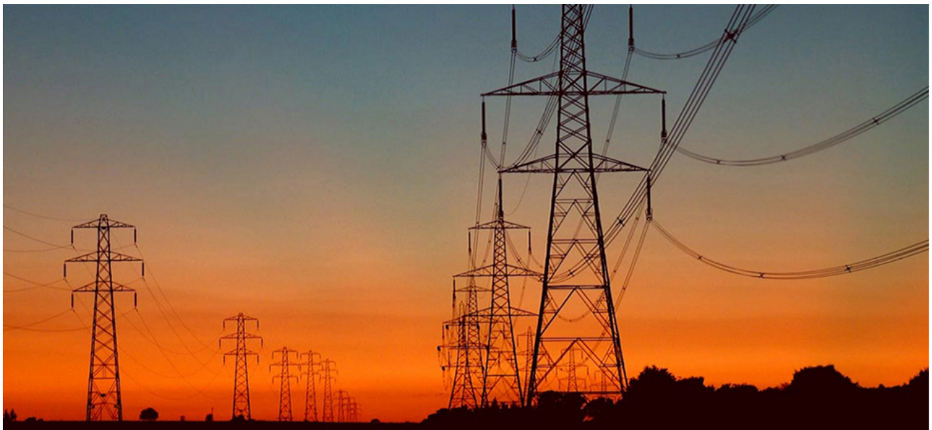
Figure 12.0.1 The current we draw into our houses is an alternating current (ac). Power lines transmit ac to our neighbourhoods, where local power stations and transformers distribute it to our homes. In this chapter, we discuss how a transformer works and how it allows us to transmit power at very high voltages and minimal heating losses across the lines.
