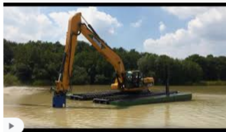
Floating Amphibious Excavator Waterking ... youtube.com
