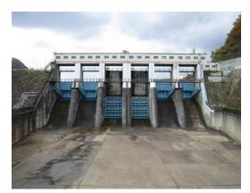
**3. Headworks:** The headworks consist of the diversion structures at the head of an intake. They generally include booms and racks for diverting floating debris, sluices for by-passing debris and sediments and valves for controlling the flow of water to the turbine. The flow of water into and through headworks should be as smooth as possible to avoid head loss and cavitations. For this purpose, it is necessary to avoid sharp corners and abrupt contractions or enlargements.
