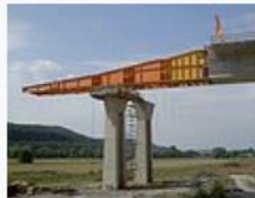
Autobahn A73 Itz Valley, Germany
