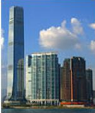
ICC tower, Hong Kong 484m 2010
