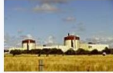
Ringhals nuclear plant Videbergshamn, Sweden
