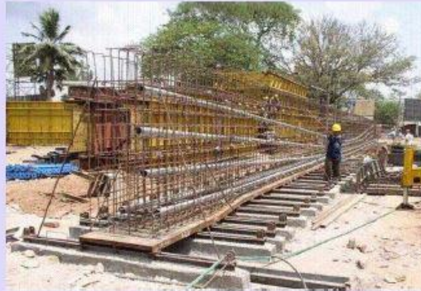
(a) Fabrication of reinforcement
