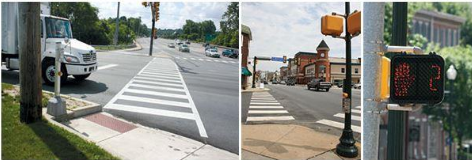
A high-visibility crosswalk at the intersection of US Route 30 Business and PA Route 100 in West Whiteland Township; A high-visibility crosswalk in Downingtown Borough; A countdown timer in West Chester Borough.
