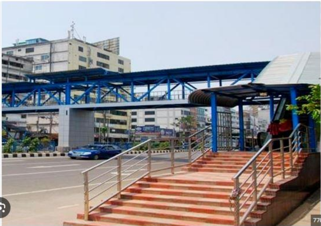
Escalator Foot Over Bridge - Projects - MAQ Engineering Ltd.
