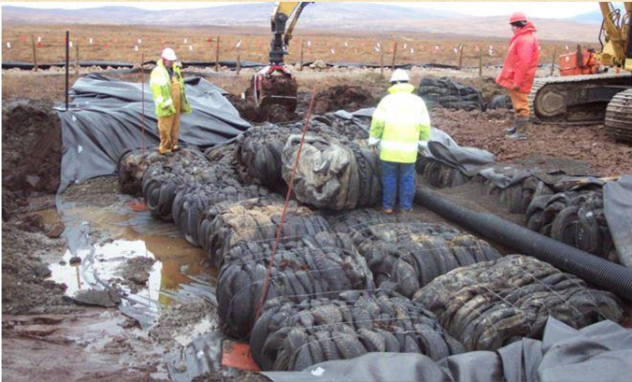
Recycled materials can also be used in road construction.
