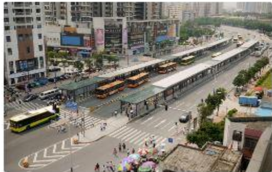
Fig. 24.49 Dongpu BRT station in Guangzhou (see layout at Figure 24.45) provides at-grade station access at both ends, combined with mixed-traffic U-turns. Karl Fjellstrom.
