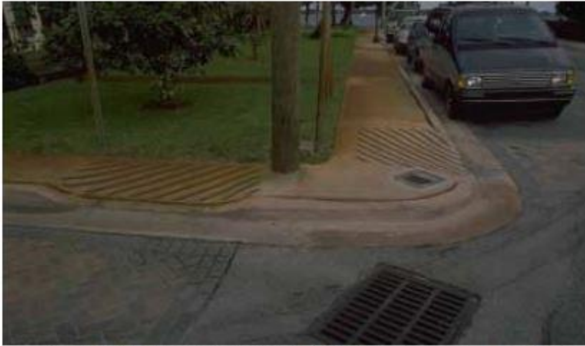
A 7-foot radius allows for a slow and safe turn. As the radius increases, so does the speed of the vehicle.
