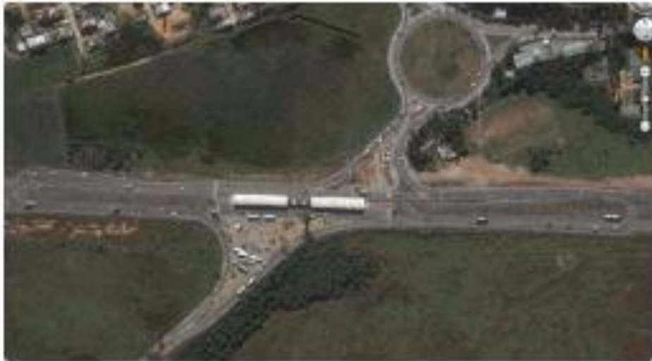
Fig. 24.48 Traffic is diverted past this TransOeste station in Rio de Janeiro before it is allowed to perform U-turns away from the station. Google Earth.
