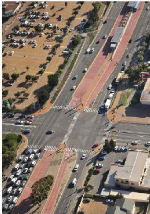
Fig. 24.29 Cape Town, South Africa's standard four-phase intersection with a cross-traffic-turn waiting area using the narrowed width of the opposite way. Bruce Sutherland .
