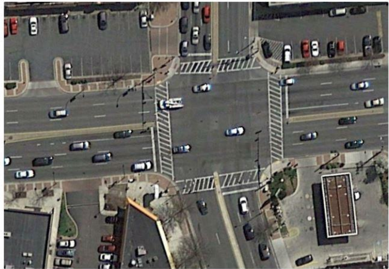
Fig. 24.30 Lanes as narrow as 2.4 meters are an effective way to improve intersection capacity, as in this intersection in Montgomery County, Maryland, USA. Google Earth .
