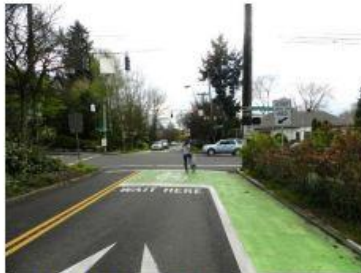
Bicycle boulevard with bike box intersection (Credit: Toole Design Group)
