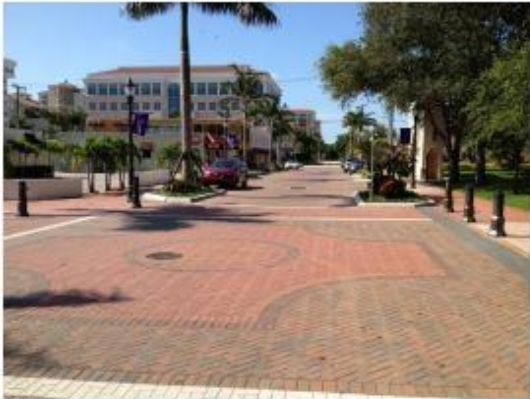
Festival street with flush sidewalks separated by bollards (Credit: Kimley-Horn and Associates, Inc.)
