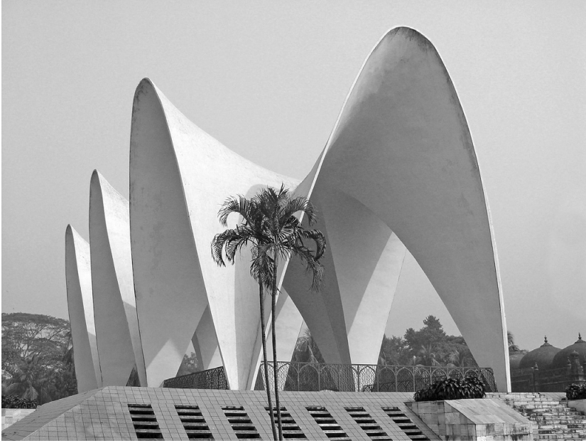
Plate 19.4. The Mausoleum of the Three Leaders (Tin Netar Mazar) in Dhaka was constructed in the 1980s. It honours three prominent politicians who were active in the early Pakistan period: A.K. Fazlul Huq (1873–1962), H.S. Suhrawardy (1892–1963) and Khwaja Nazimuddin (1894–1964). The mausoleum’s architect was S.A.K. Masud Ahmed. A Mughal-era mosque can be seen in the background.
