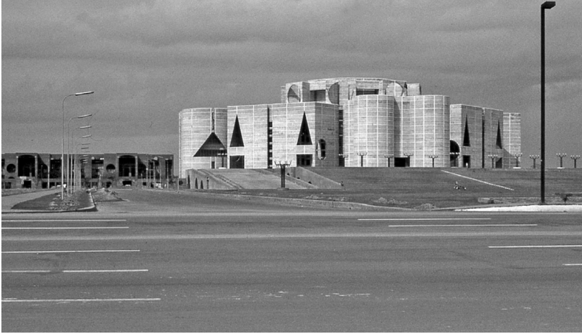
Plate 11.4. The Bangladesh Parliament, originally conceived as Pakistan's National Assembly Building. Designed by Louis Kahn in 1962, it was completed in 1983.
