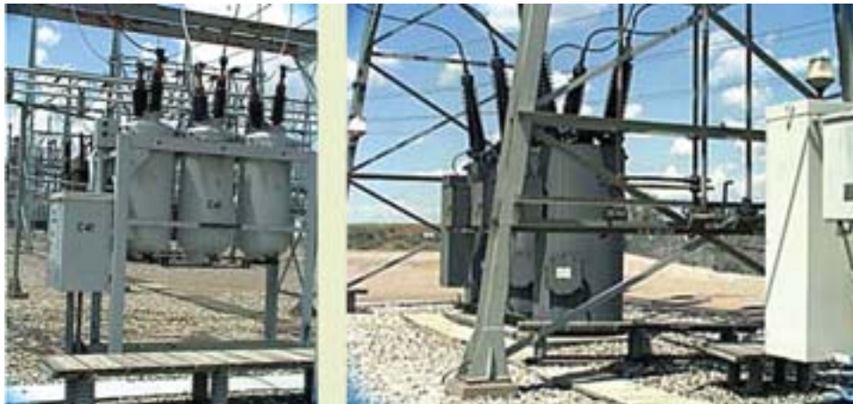
Oil Circuit Breakers
