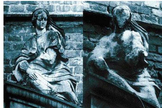
How acid rain affects stonework. The picture on the left was taken in 1908. The picture on the right was taken in 1968
