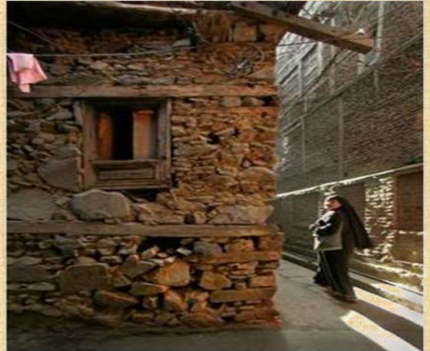
An historic house of Taq construction still extant in Srinagar, Kashmir, India.
