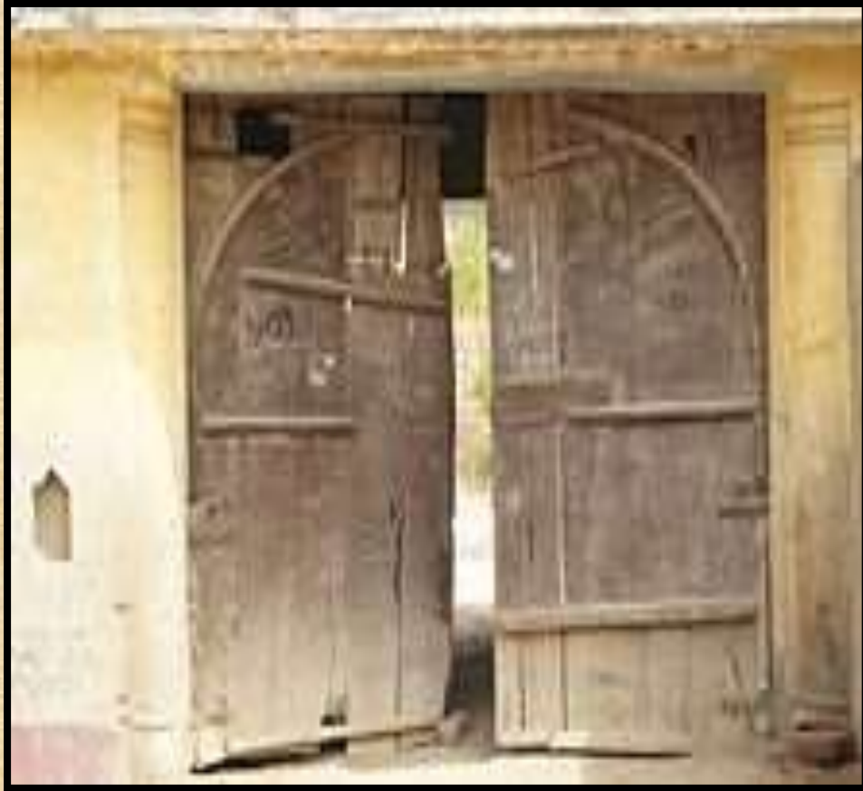
Timber compound gate in Punjab Made of wooden planks
