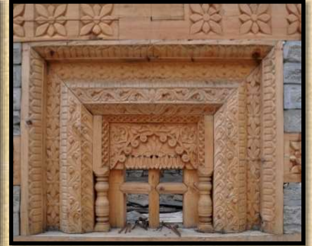
Windows in dhajji wall construction in Himachal Pradesh
