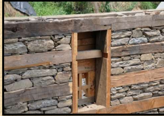
Windows in dhajji wall construction in Himachal Pradesh
