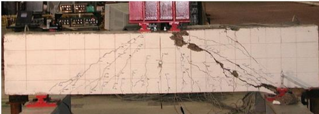
Inclined cracks are formed due to shear, which are known as shear crack
